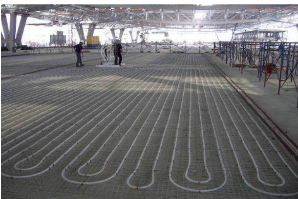
Figure 6 Radiant floor cooling system in construction
